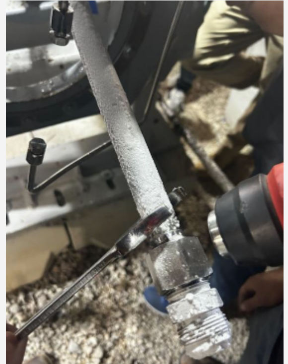
Image: Heating up fitting post-cold-flow to disassemble
