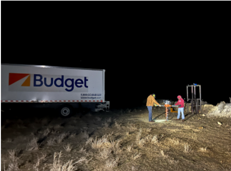
Image: Digging to set concrete anchors for lift infrastructure
