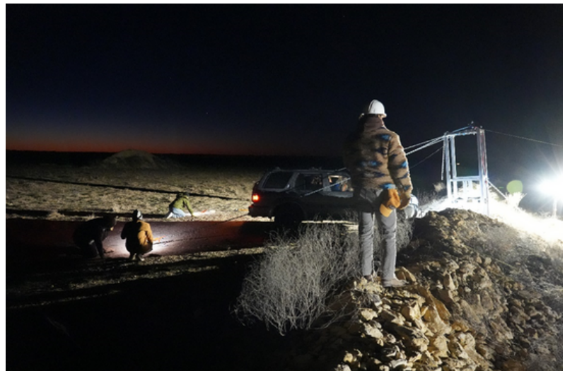
Image: Mason Nothaft overseeing lift operations
